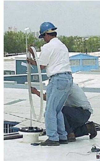
6. After the float and weight are in the tank, thread bushing into tank or bolt flange into position.
